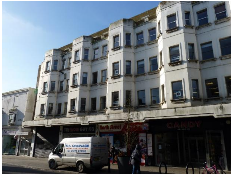
Nos.21-25 North Street
