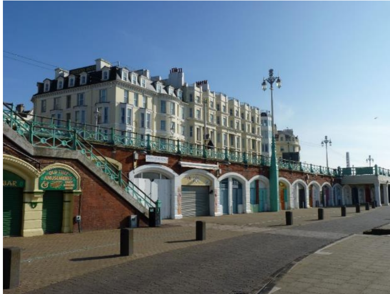
Brick arches supporting King's Road
