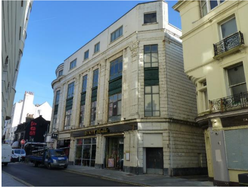
Entrance front of the former ABC Cinema on East Street
